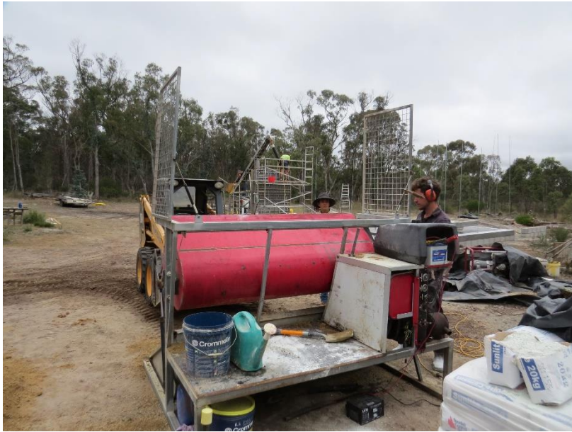
A bobcat is used to transfer the mixed deco from the mixer to a conveyor belt which delivers the soil to the formwork.
