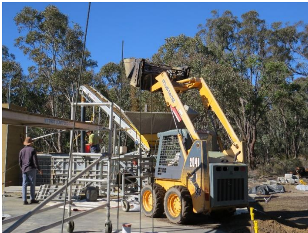
The deco is then rammed using a pneumatic stick rammer powered by an air compressor.
